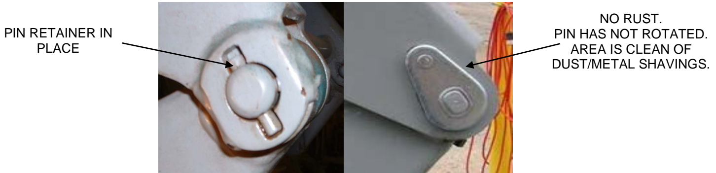
Figure 2: Scissor end pin connection - no evidence of damage
